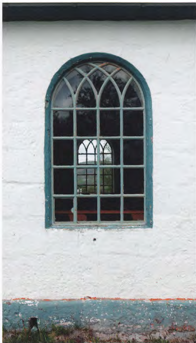
8. Kirkjugluggarnir eru úr steypujárni, þeir eru í hringbogastíl en efst sveigjast gluggasprotarnir í oddboga. – The windows are round-arched, of cast-iron. At the top of the windows the glazing bars form pointed arches.
