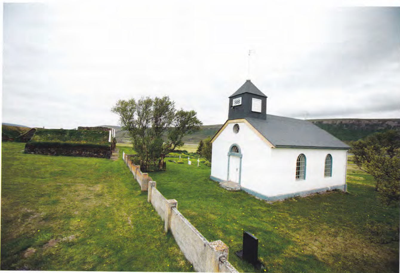
7. Þveráarkirkja sumarið 2012. Kirkjan er hlaðin úr tilhöggnu móbergi, reist á árunum 1878-1879. Kirkjubakið var upphaflega lagt þakpappa en árið 1905 var það járnvarið. Árið 2011 var settur þakpappi á turn og kirkjubak eins og verið hafði í öndverðu. Handan kirkjunnar sér í gamla bæinn á Þverá. – Þverá Church, summer 2012. The church was built in 1878-9 of blocks of cut hyaloclastite. The roof, originally covered in asphalt felt, was fitted in corrugated iron in 1905. In 2011 the tower and roof were once again covered with asphalt felt, as they were originally. Beyond the church is the old turf farmhouse.
