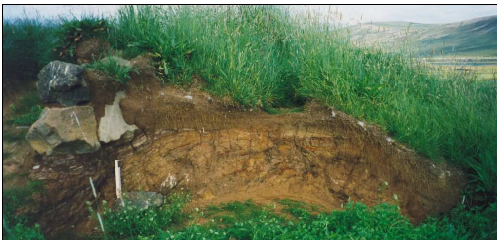
Figure 2.14 Ruined turf building of unknown age in the infield north of the house. Note the melted aspect of the turfs, which nevertheless show characteristic lenses of oxidised iron (reddish brown), decomposed organic matter (dark brown), and leached soil (very pale brown). The white scale to the left of the photograph is 20 cm long.
