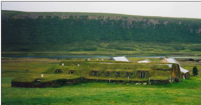
Figure 2.7 The back of the house, facing east, showing the grassy roof, from which light holes protrude. The glass windows in the bedroom and sitting room were a later addition. The low room on the left side of the house caps a small stream, and was used to keep milk cool.
