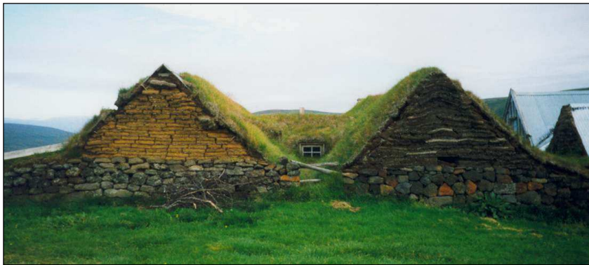
Figure 2.5 Schematic section of the kitchen at Þverá, showing the construction of the walls and roof (from Olesen & Kjær 1972, 35), and a close-up of a turf wall (left). The stripy aspect of the wall was produced by the redistribution of iron as the turf dried out.
