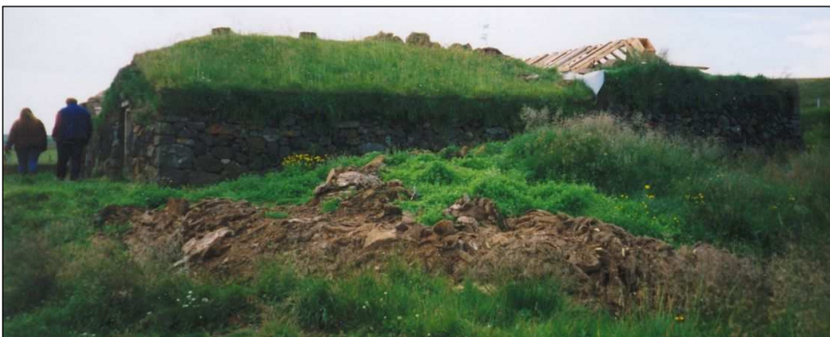
Figure 2.11 Midden heap containing fragments of turf waste that was produced during the repair of the roof of sheephouse 1.
