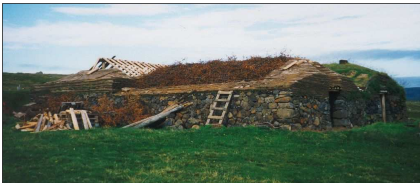
Figure 2.8 Turf roof of sheephouse 1 (right) and attached hay barn (left) undergoing repair. A mat of birch brushwood has been laid on top of the timber roof beams, in preparation for the grassy turf that will be laid on top.
