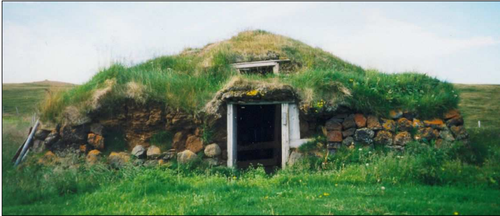
Figure 2.12 Sheephouse 2, fifty years after abandonment, with its roof still intact, but with an outer skin of stones beginning to peel away. The roof began to collapse two years after this photograph was taken.
